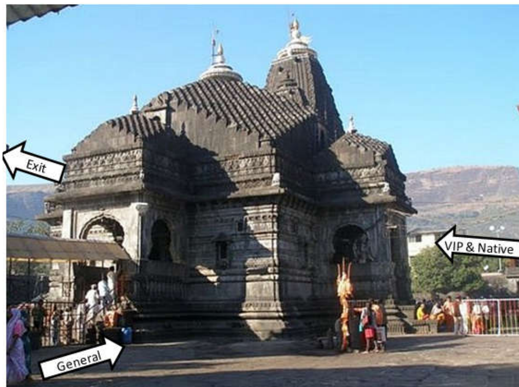
Figure 2: Entry and Exit doors to the temple
